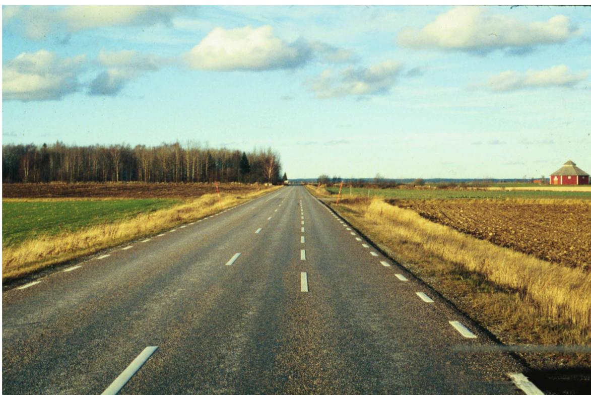
*Figure B.2 - Broken line: 3 + 3 m; width: 10 cm*
