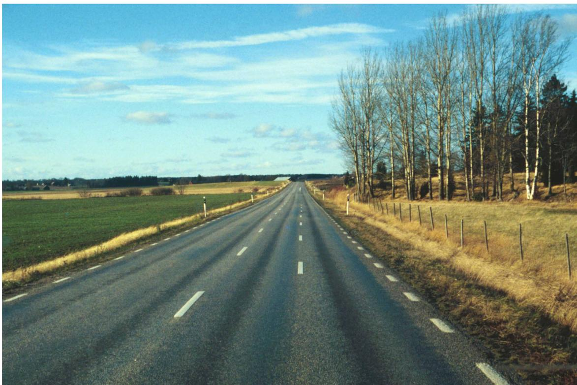
*Figure B.1 - Broken line: 3 + 9 m; width: 10 cm*
